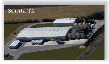
Just outside of San Antonio, TX, the Schertz facility rests on 14 acres strategically located off Interstate 35, a north-south highway that spans the US. Our 80,000 sq ft lube plant has an external tank farm that can hold 2 million gallons. Our newest structure, a 25,000 sq ft grease plant, houses 14 kettles including a Stratco contactor and produces an annual throughput capacity in excess of 30 million pounds. Our QC lab tests all incoming and outgoing raw materials and finished products.
